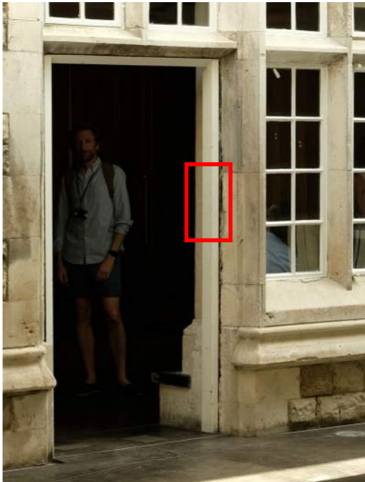
Existing condition of window to Tower Bridge Arch 01 with steel portal frame partially concealing damaged stonework
