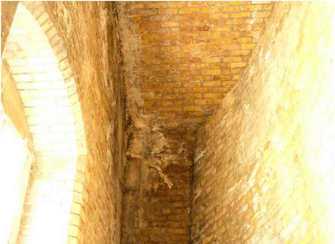
Spalling, cracking and efflorescence and staining to brickwork internally
