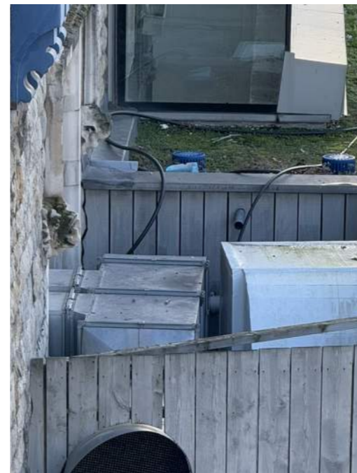
Existing condition of window to Tower Bridge Arch 02 with removed glazing and MEP ductwork penetrations
