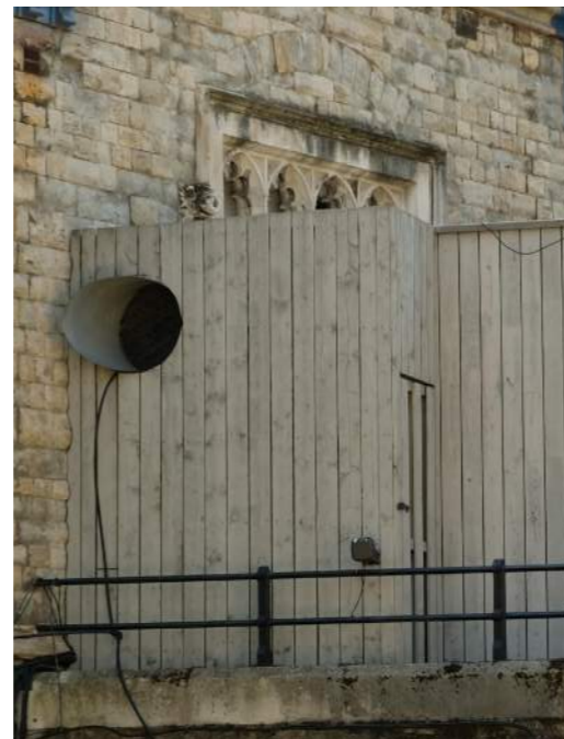
Existing condition of window to Tower Bridge Arch 02 with removed glazing and MEP ductwork penetrations
