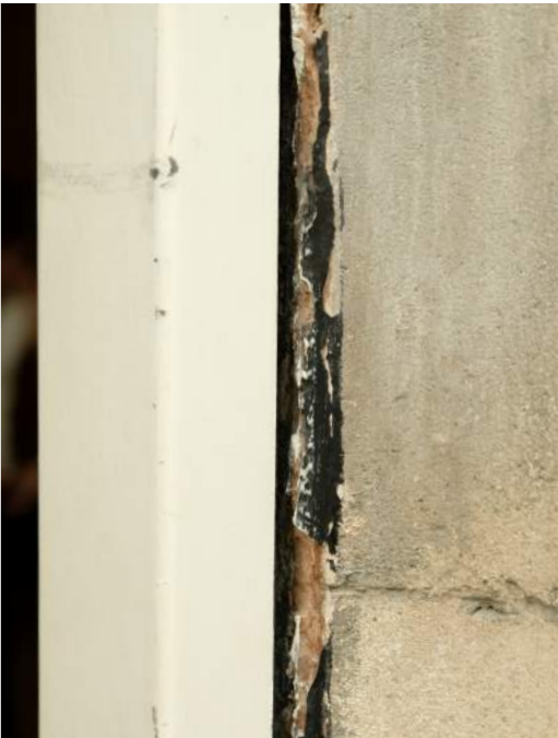
Existing condition of window to Tower Bridge Arch 01 with steel portal frame partially concealing damaged stonework
