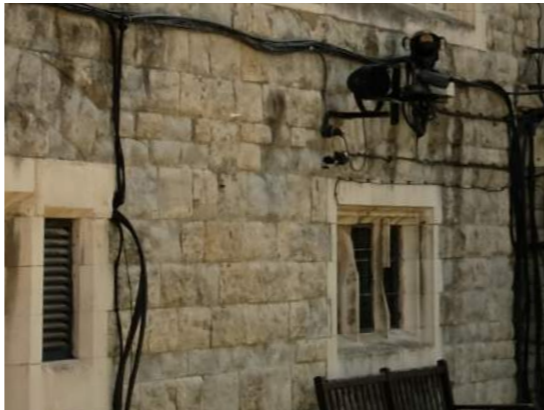
Detrimental modern louvres, lighting and cabling
