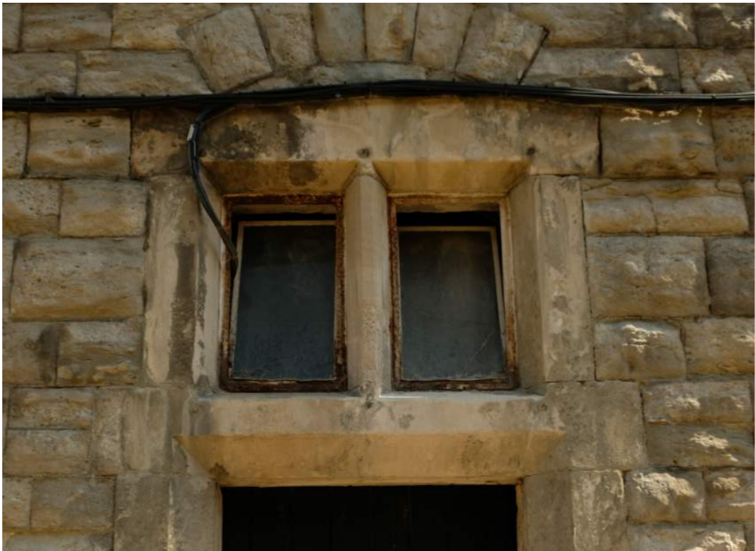
Existing poor condition of external masonry and corroded and failing windows
