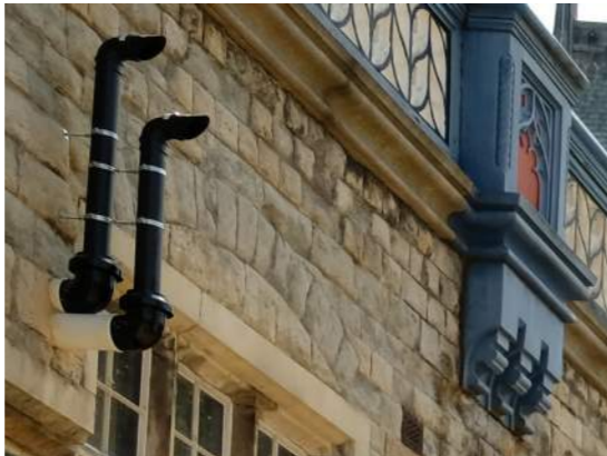
Detrimental modern pipework
